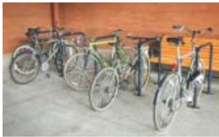
*Adequately spaced bike racks, with 30 to 36 inches between racks, allow obstacle-free access to bike parking spaces.*
