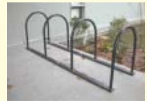
*The inverted-U bike rack, whether as stand-alone units or on rails with multiple Us, make for excellent bike parking when the inverted Us are spaced at least 30 inches apart. Two bikes can use each inverted U.*
